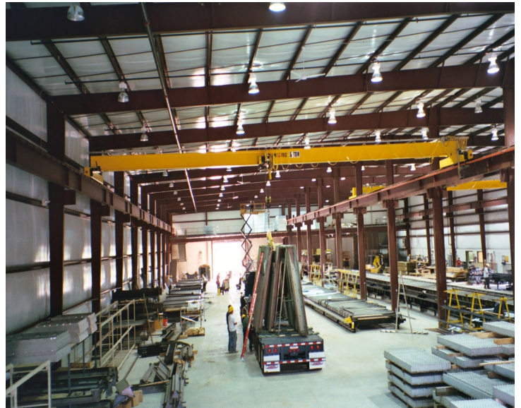
Crane-Tec cranes in use after completion.
