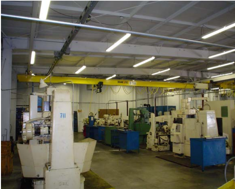
Finished product - 1 ton building supported system
